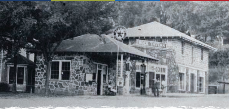
George M. Reed Building
