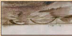
Old Roubidoux Bridge is visible between center arch, circa 1923
